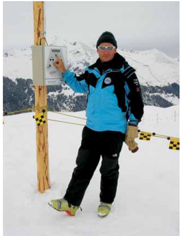
Permanently installed control unit
